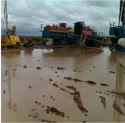
BWP 39 at Blackwater CSG Field
