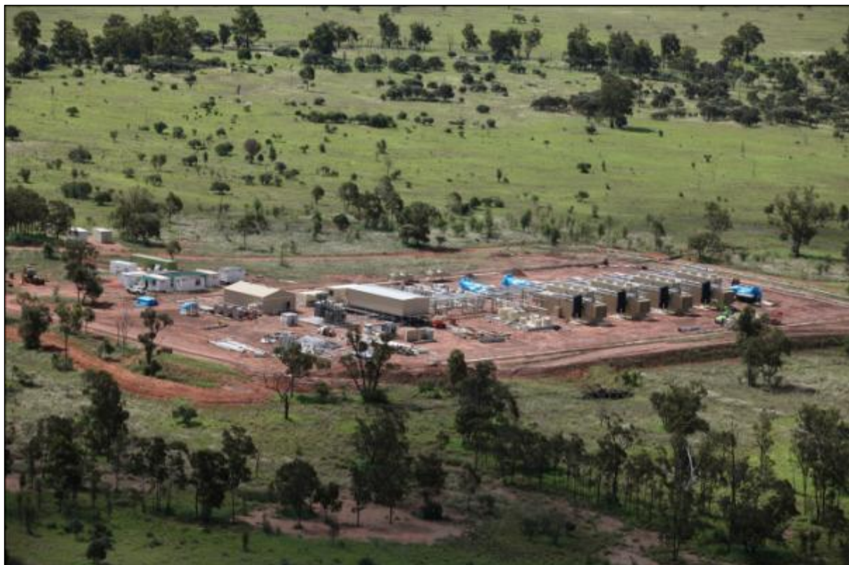
Aerial View of Construction Site for Blackwater Power Project (Jan 2011)
