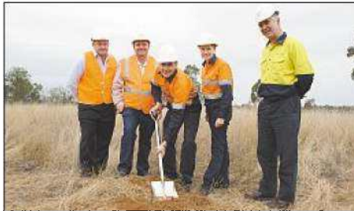
■ TURNING THE FIRST SOD: Bow Energy's John De Stefani (centre) was joined by Mayor Peter Maguire to officially mark the commencement of the Blackwater Power Project.
