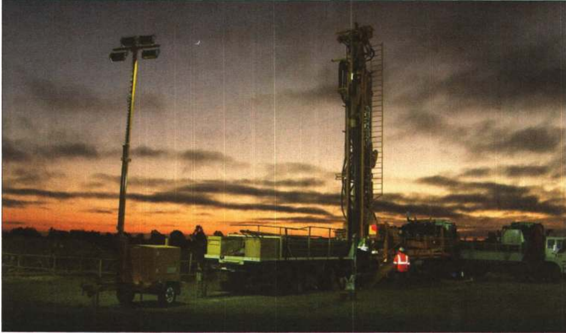
RS Depco Rig 28 on hole BW-2a at dawn
