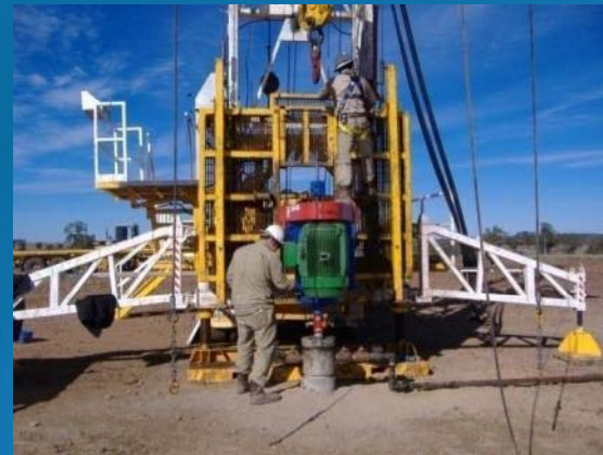
Installing an electric drive head
